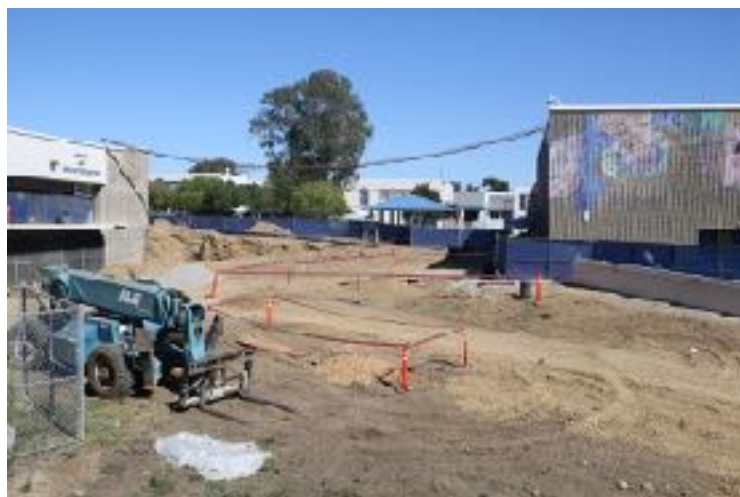
Construction at SDHS, LaBella Photography, 2023, SDHS Alumni
