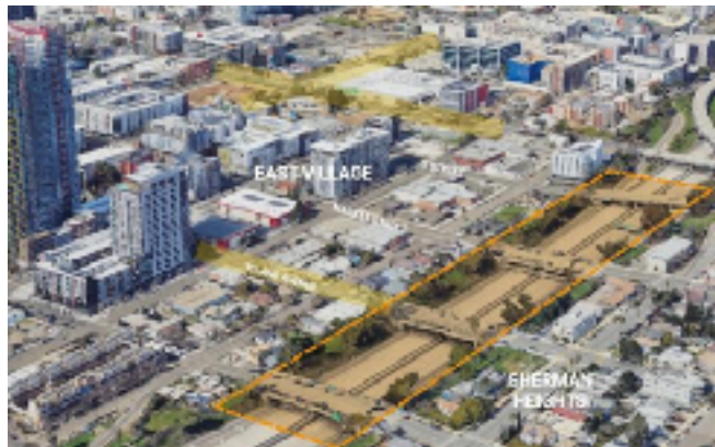
I-5 lid locations: top, 6th Ave.-Park Blvd., bottom, G-J streets., San Diego Commons and Urban Division Story Map, 2023
